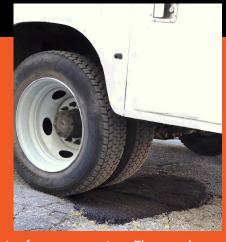
Tip: Need Faster Hardening? Apply a thin layer of Portland Cement to the top of the repair after compaction. The patch should then be compacted one more time to harden the surface.
